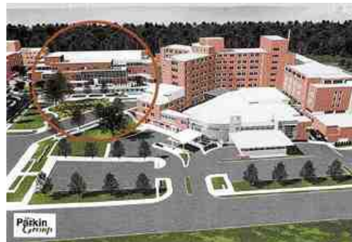
The Grand River Regional Cancer Centre (circled), now under construction at Grand River Hospital on King Street West in Kitchener, will include the J. Wesley Graham Family and Patient Resource Centre, where cancer patients and their families can use books, articles and the Internet to find information about cancer. (The Parkin Group Architects)
